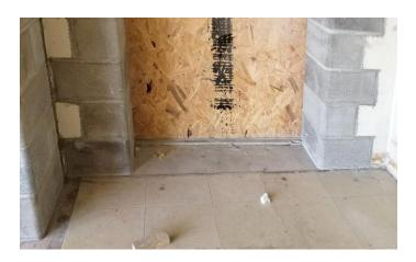
Masonry contractor cuts and preps two openings into the existing brick walls. The new interior opening is boarded up. Opening dimensions are always guaranteed or verified in field prior to manufacturing to ensure a quality fit.
