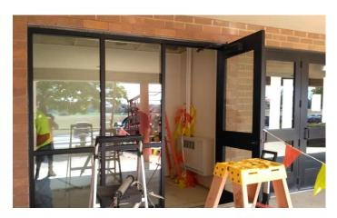
Capitol installed the prefabricated storefront framing first. Then, the new Capitol wide stile doors are installed along with all remaining door hardware. All laminated Low-"E" insulated glass units are then glazed into the doors and framing.
